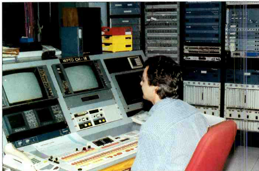
One of the master control stations used at GDPT. The routers and automation units are in the racks in the background.
