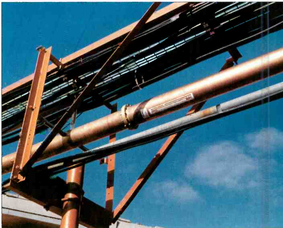
Both rigid coaxial line and semiflexible coaxial cable are included in this transmission line installation at WGTW (Channel 29), Traverse City, MI.
